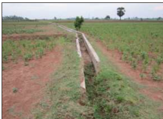
Plate 4: Concrete drains for irrigation
